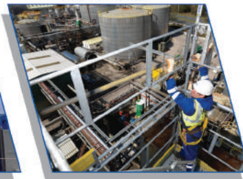
PROCESS, MECHANICAL & ELECTRICAL
